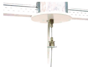
Drop ceiling J-Box for feed locations makes for a easy code compliant installation.
