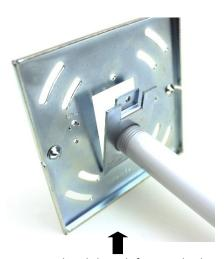
Insert Tail End then shift tapped side on inside of crossbar and fasten with 8/32" screw
